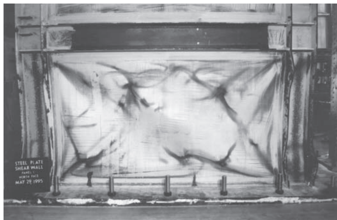
Fig. 8. First story of Driver's SPSW (photo courtesy of R.G. Driver).
